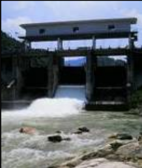
Huaiji, Guangdong 105.6MW hydro (88.6MW in operation)
