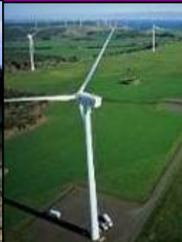
Woolnorth Bluff Point, Australia* 65MW wind
